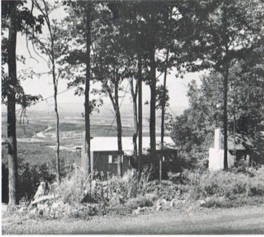
Sturdy masonry for year-around living, overlooking the Shenandoah.
