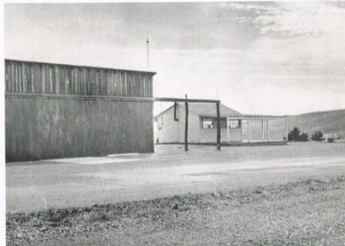
Property Office and equipment building at Skyland Estates.
